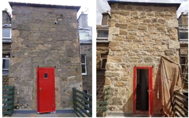
Fig 23 and 24. West stair wall before and after
