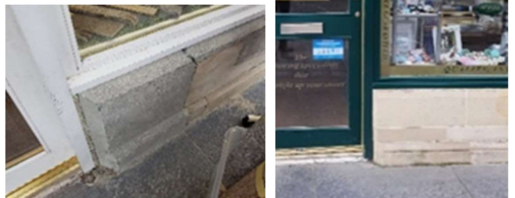
Fig 27 and 28. Concrete infill and ashlar reconstruction
