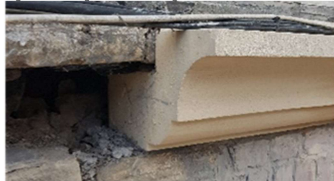
Fig 7. Reconstructed cornice during
