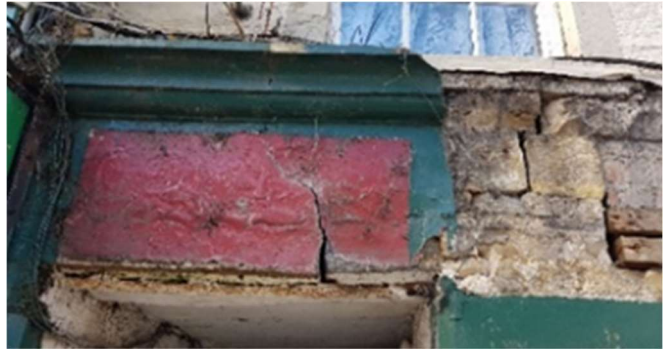
Fig 6. Existing cornice during works
