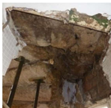
Fig 19 and 20. WC unsupported recess and brick infill
