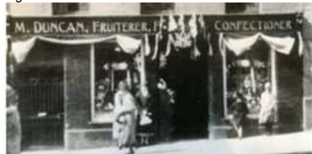
Fig 2. Shop front pre alterations, note gate
