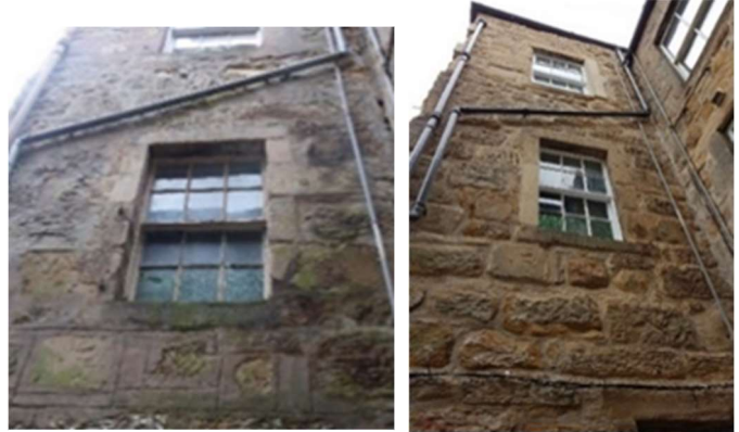
Fig 25 and 26. South stair wall before and after
