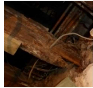
Fig 14 and 15. Dry rot staining, timber decay
