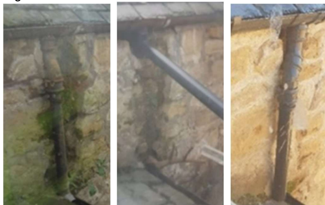
Fig 10 and 11. RW goods before during and after works
