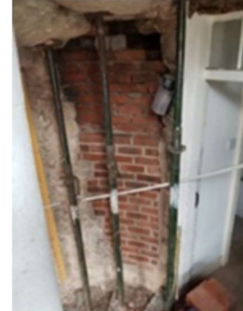
Fig 19 and 20. WC unsupported recess and brick infill
