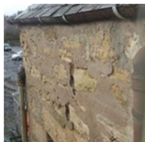
Fig 16 and 17 Existing cement pointing, dry rot works
