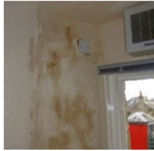
Fig 14 and 15. Dry rot staining, timber decay
