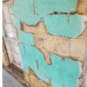
Fig 18 and 19. Paint removal, masonry tooling
