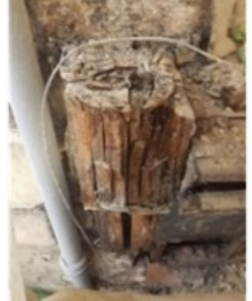
Fig 12 and 13. LH console bracket before and during works
