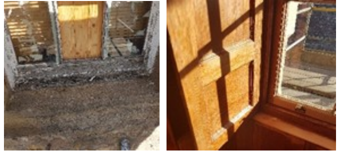
Fig 20 and 21. Window before and after repair
