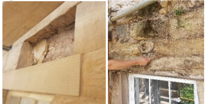
Fig 22 and 23. Stone indent and vegetation removal
