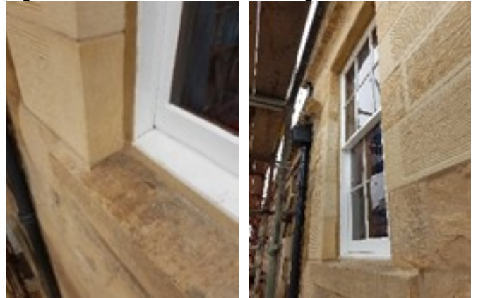
Fig 24 and 25. Front window after works
