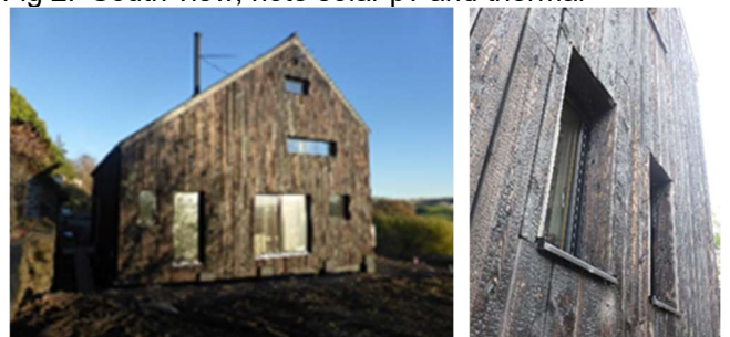
Fig 3 and 4 East view and cladding detail
