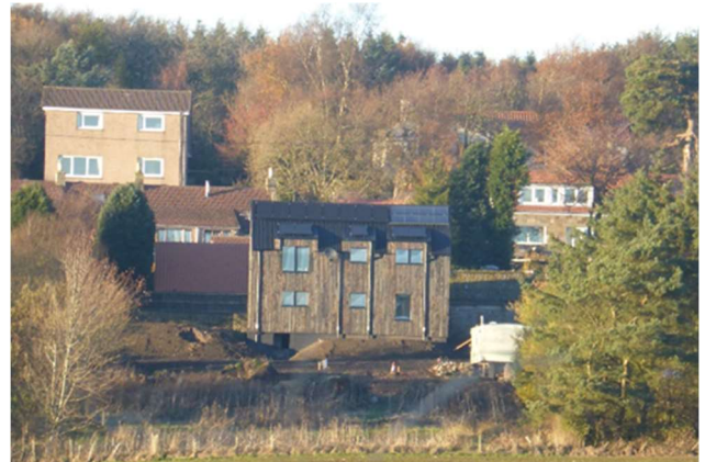
Figure 1. House viewed from South
