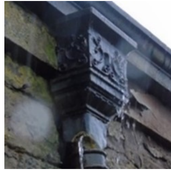
Fig 23 and 24. Failed rainwater goods, cement pointing
