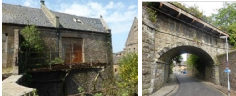
Fig 14 and 15. Warehouse 5 and 6, former rail bridge
