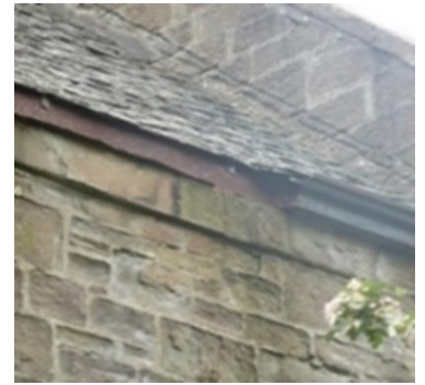
Fig 23 and 24. Failed rainwater goods, cement pointing
